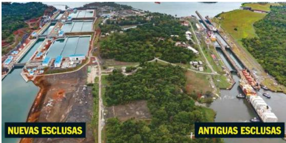
Comparison of the new 2016 locks in Panama to the previous ones opened Taken from: Semana Magazine 6/4/2016 "Panama Canal Expansion Ready"
